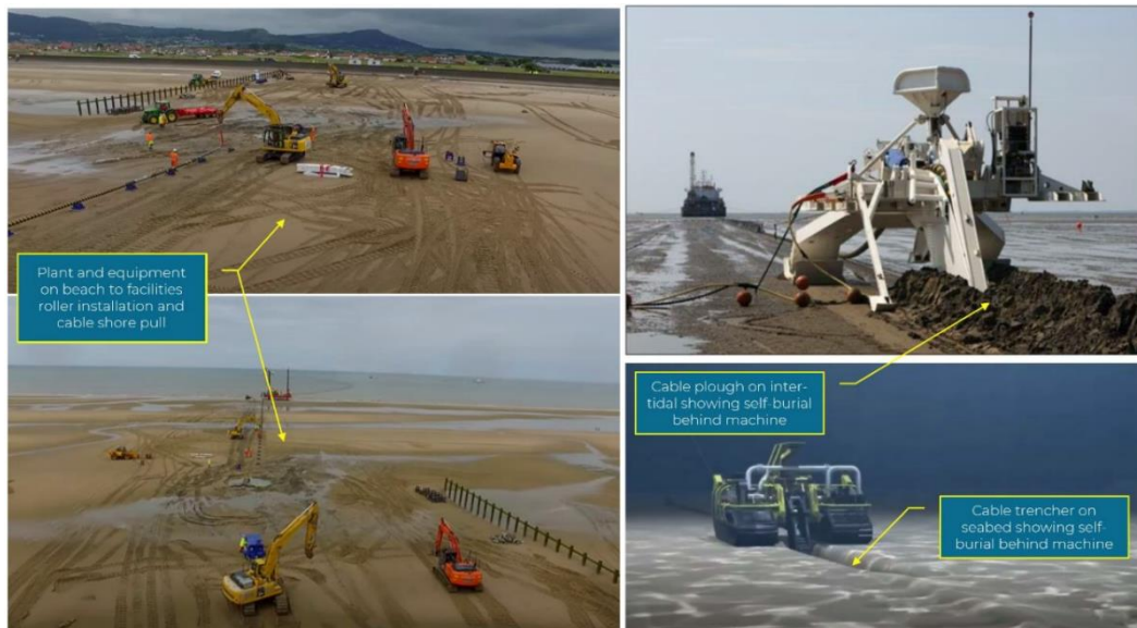
Figure 3 2- Typical plant and equipment for cable installation across inter-tidal similar to offshore wind farm cables historically installed between Prestatyn and Rhyl.
